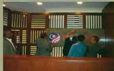
Putting up MPI signage
